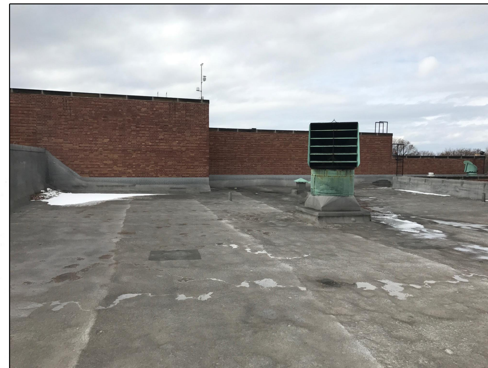
FLAT ROOF AREA FOR EXTERIOR MECHANICAL EQUIPMENT
